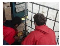
Then a tube connection is made on the outside. (Materials needed: Connector  $\frac{1}{2}$ ", Male gas adapter  $\frac{1}{2}$ ")
