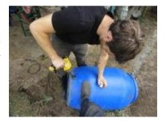
The next step is constructing a hose connection. (Materials needed: PVC Tank connector 1", Tap PVC 1", Adapter pipe to hose 1")
