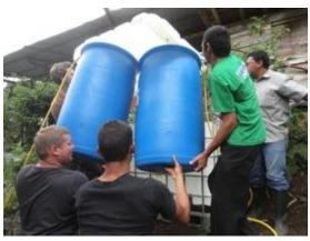
The 1000 liter container is then filled with water, and chlorine added to prevent mosquitos. Rocks are placed on the lid of the gasholder, weighing it down, creating more gas pressure. This can be seen in the opposite picture, between the two blue containers. The number of rocks and thus the weight depends on the type of stove used, the length and diameter of the gas tube and other factors. The optimal weight is best calculated through trial and error.
